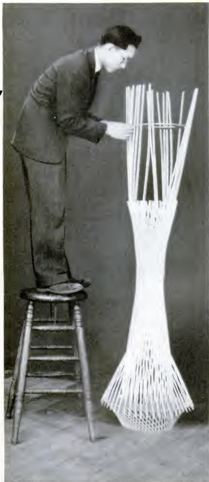
A student of industrial design building a complicated structure of soda straws. Toothpicks form the joints
